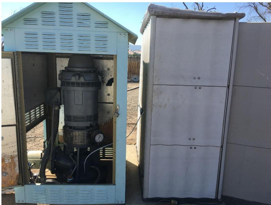
**Figure 1. Station 2 Well – Well Injection Piping**
