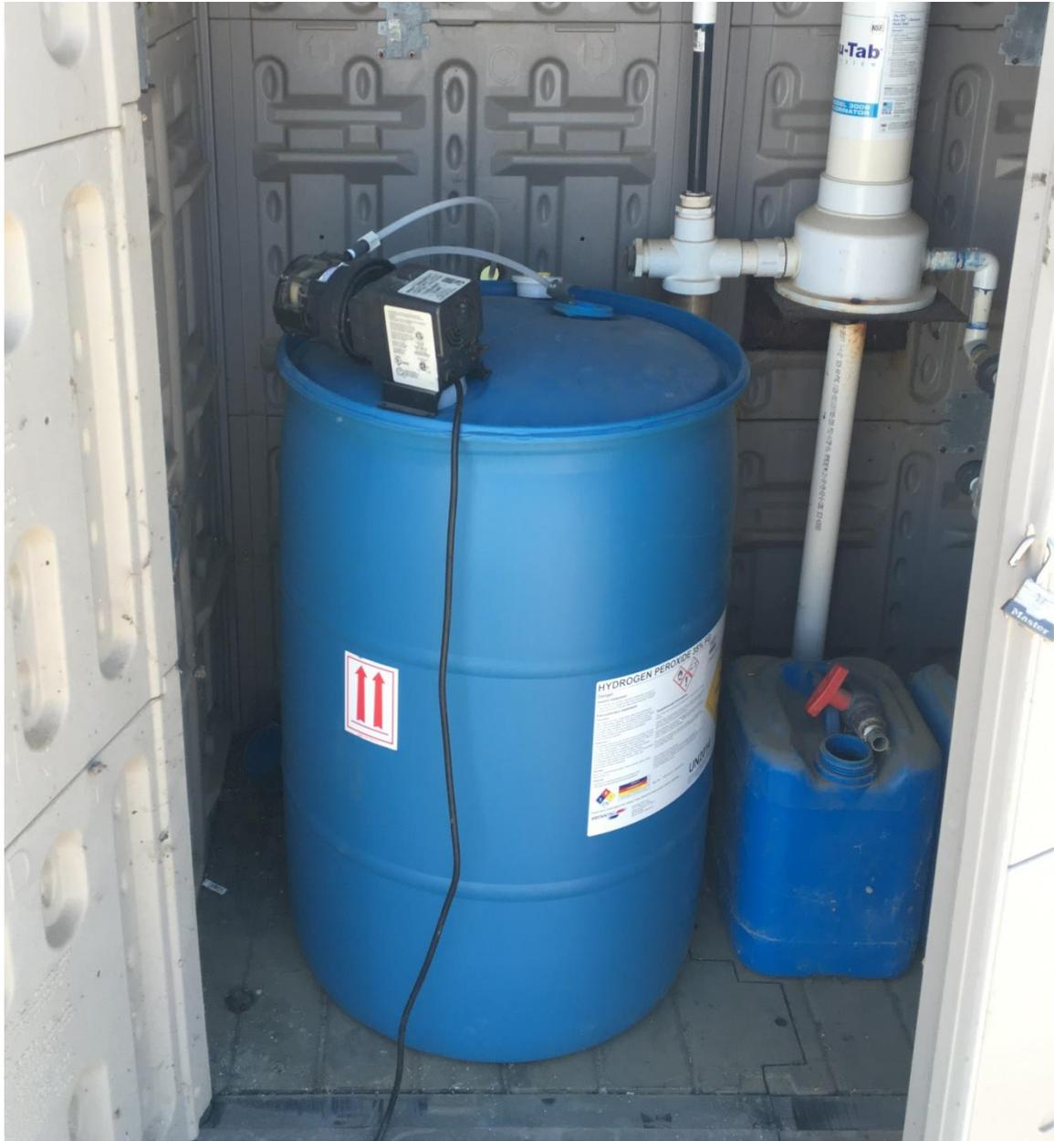
**Figure 2. Hydrogen Peroxide Container and Injection Pump**
